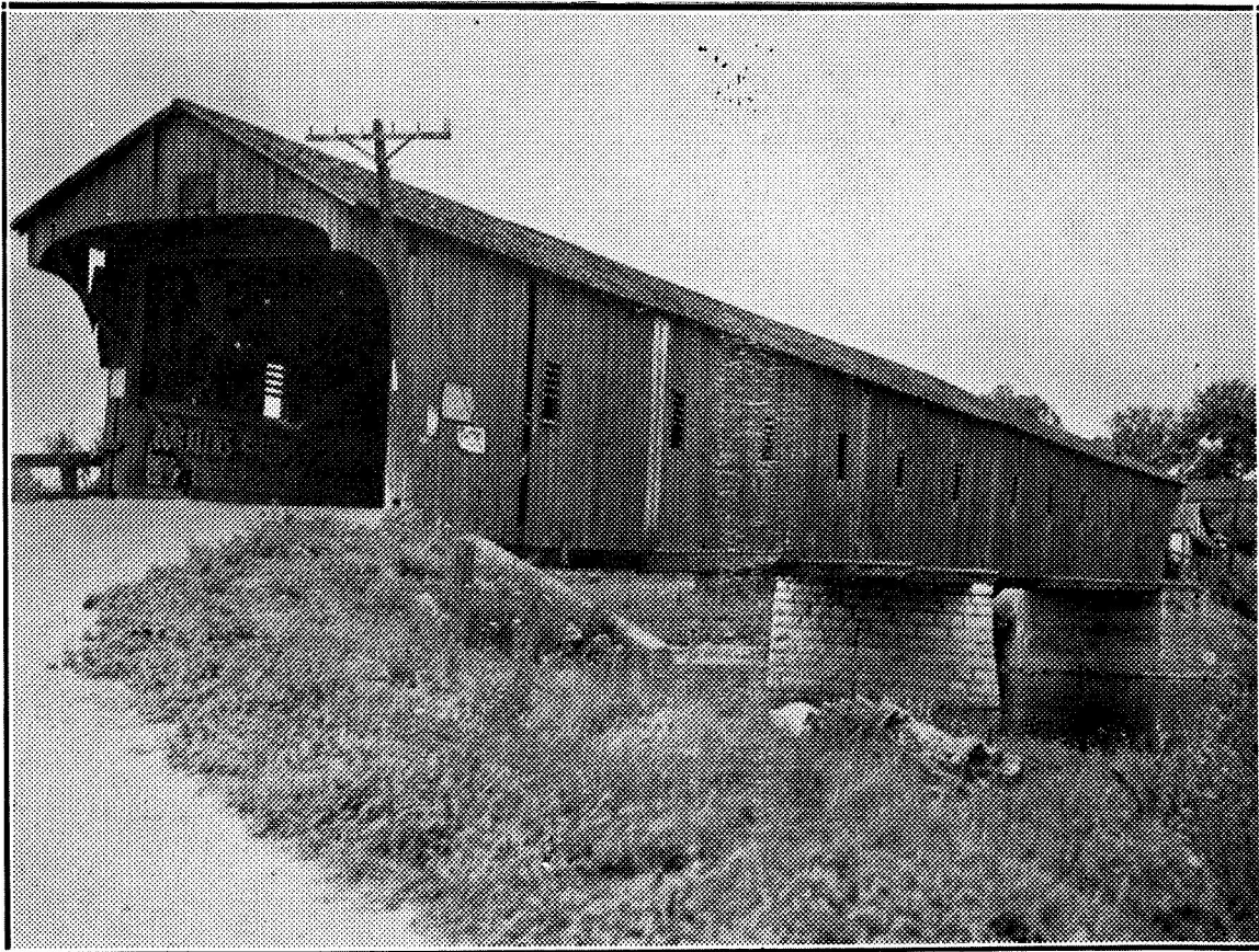
Covered bridge at West Montrose, said to be the only one of its kind remaining in Ontario. Built, as nearly as can be ascertained, in 1881 by Benjamin Bear, a builder and contractor who lived near Doon. The bridge consists of two 90-foot spans and has an inside width of 17 feet.
